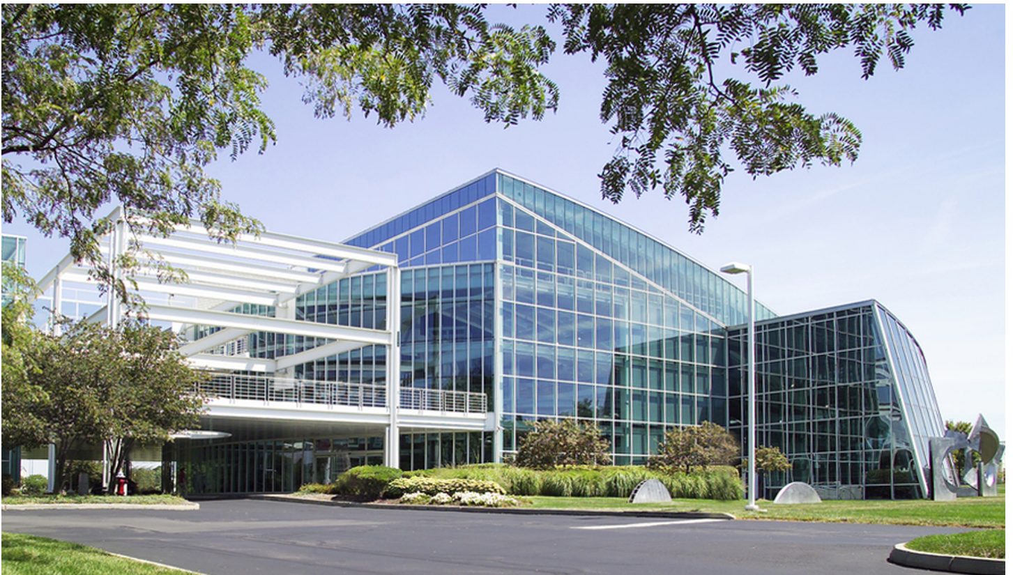
Top Left, Clockwise: 1. Trinity Episcopal Cathedral; Charles F. Schweinfurth, 1907 2. Ohio Aerospace Institute; Richard Fleischman Architects, 1993
